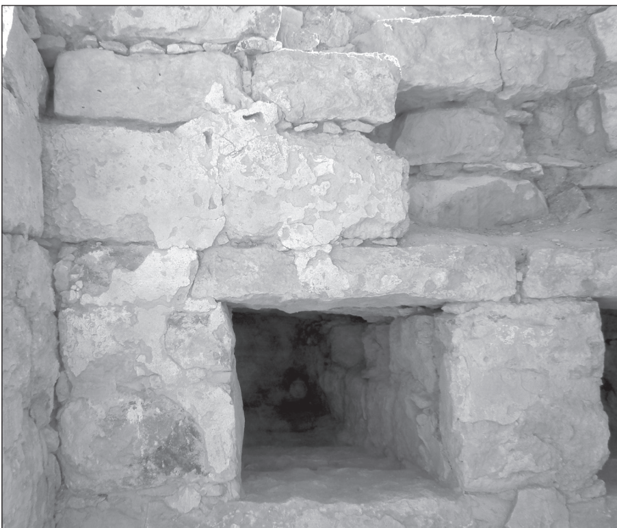
9. Surviving plaster on the south-east wall of PHTP Tomb 10 ( Photo by L. Wadeson ).
